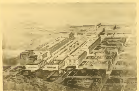
XXVIII. CLEVELAND GROUP PLAN. View looking towards the Lake from the proposed civic center.
